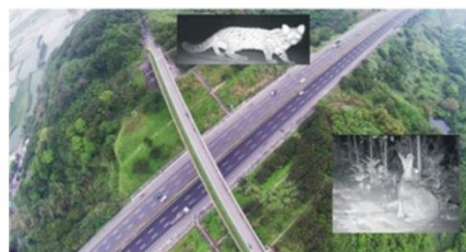
Image : Multifunctional across bridge of Tung-Shiau No. 1 and Taiwan hare and tigers using the channel.
